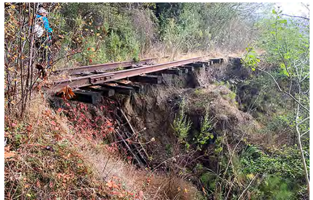
Figure 2.4.2-2 Sink Undercutting the Rail Corridor at MP 211
