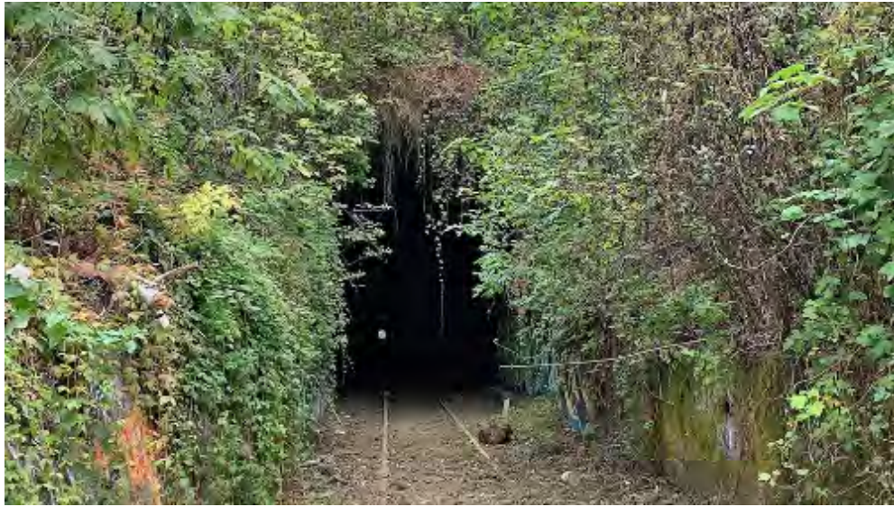
Figure 2.3.1-3 Generally Intact 1,950-foot Loleta Tunnel
