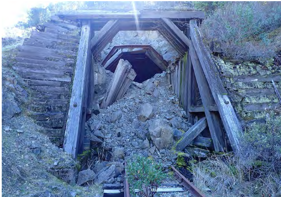
Figure 2.3.1-4 Partially Collapsed Tunnel in Eel River Canyon
