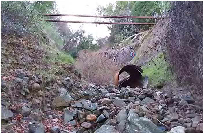
Figure 2.3.1-5 Washed-out Culvert
