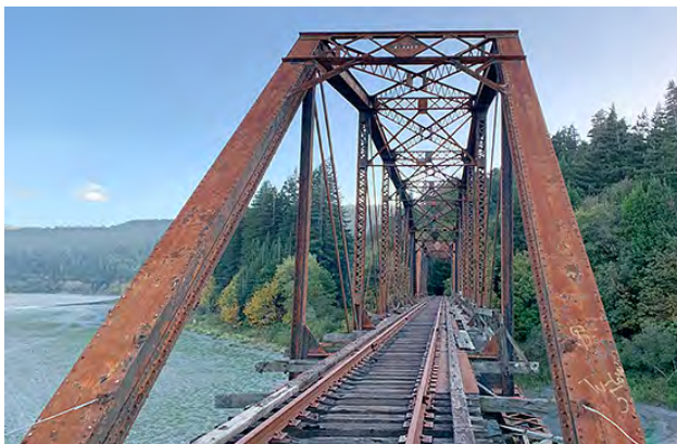
Figure 3.1.2-2 Bridge with Collapsed Decking and Condition Rating -2
