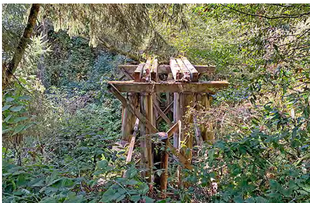
Figure 3.1.2-3 Collapsed Bridge with Condition Rating -3
