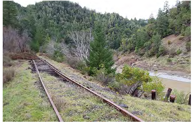
Figure 2.4.2-2 Sink Undercutting the Rail Corridor at MP 211
